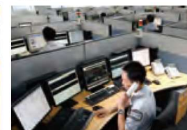
SECOM control center
