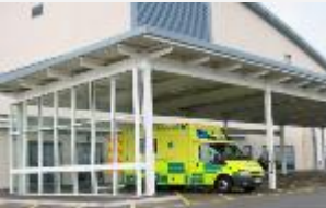
Blackburn Hospital, UK
